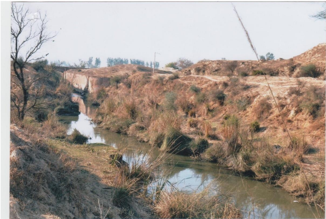
Position before laying pipeline
